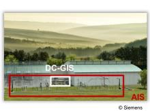
Space-saving installation, aesthetic planning, independent from environmental conditions, no fire hazard
